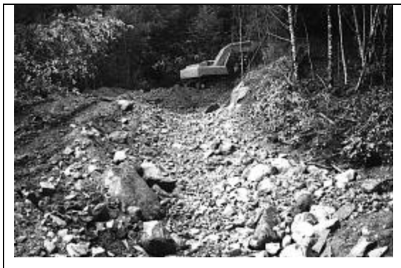
Figure 2 Re-establishment of historic channel into slide track
