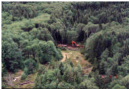
Figure 2, Aerial of dry pond sites and construction of core of lower dam
