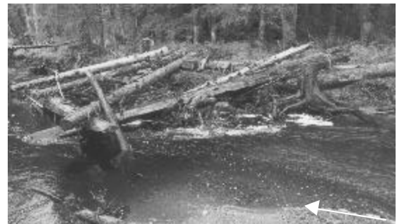
Instream: Typical A-frame LWD Structure, December 2001
