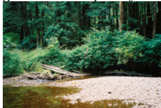
Typical constructed LWD spur during low flow.
