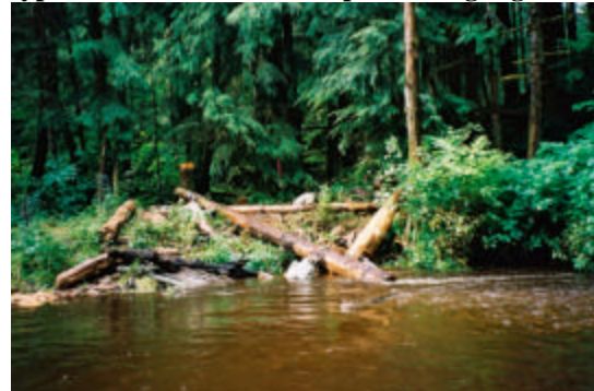
Typical constructed LWD spur during high flow.
